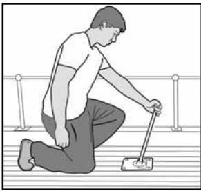
Fig. 1 Through deck installation
